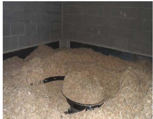
Large pellet boilers and storage bins are Dual Fuel: set up to efficiently burn either PDCs or wood pellets.
